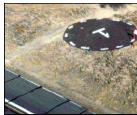
As viewed from the pattern, the wind tee is clearly defined and reliable since the maintenance.
